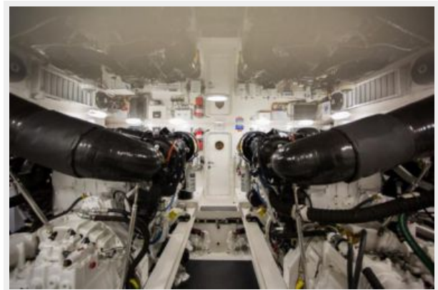
Engine Room Access to Crew Stateroom
