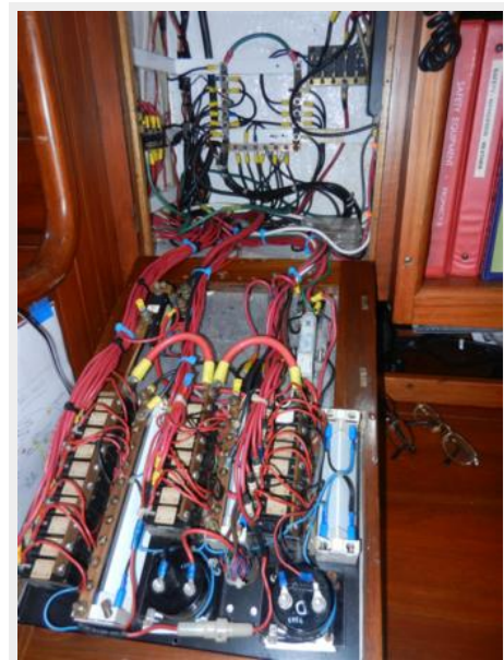
New wiring in panel
