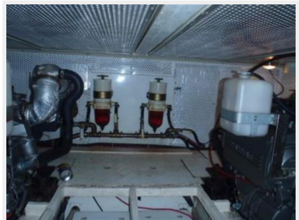
Engine room aft
