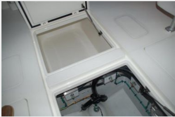
Aft underdeck bilge access
