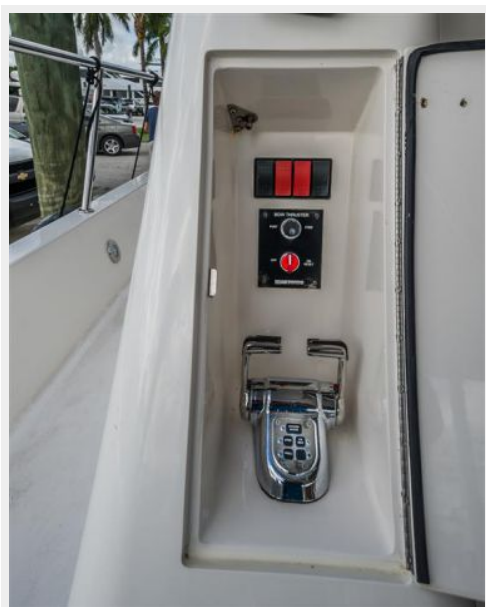
Aft Deck Controls
