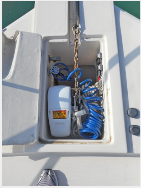
Windlass Locker-Lewmar windlass, fresh & raw water washdowns, 50 amp shore power connection
