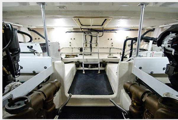
Engine Room Looking aft
