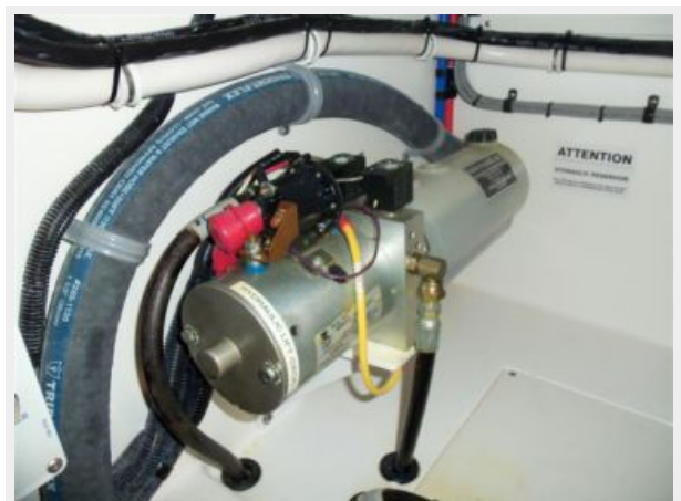
Hydraulic Hatch Mechanism
