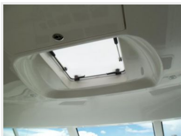
Helm Deck Vent Hatch
