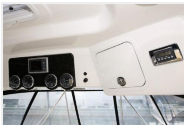
Engine Monitoring System/Bridge A/C Thermostat
