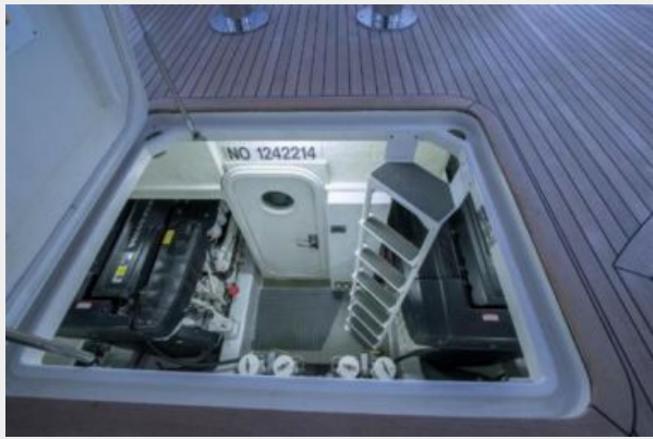
Engine Room Access
