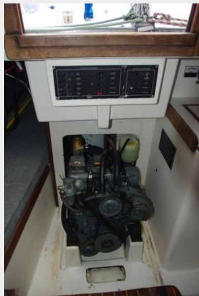
Engine box (exposed)
