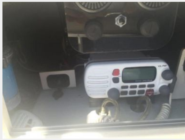
VHF in Tower
