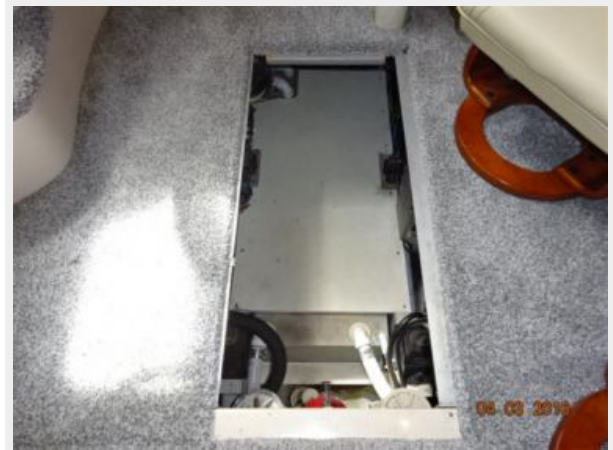
37' Mainship engine room access
