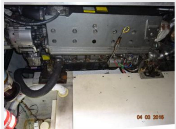
37' Mainship starboard main engine
