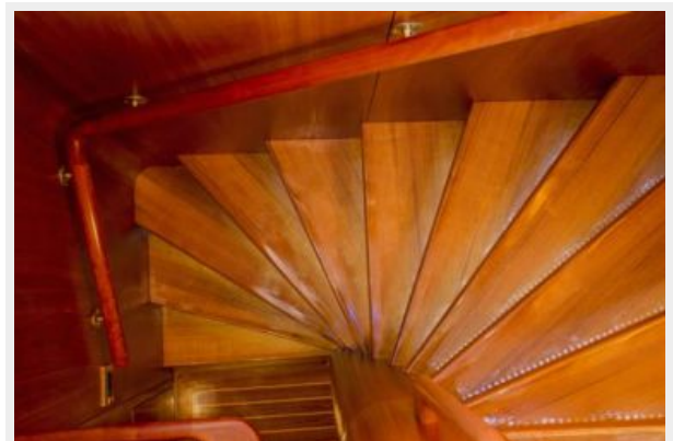
New Teak Stairways
