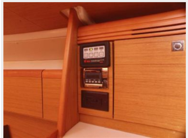
Galley A/C Control and Propane Control
