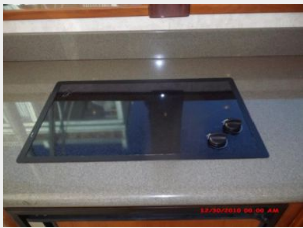
Galley 2 - Stove Top
