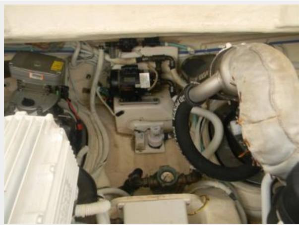
Engine Room Aft
