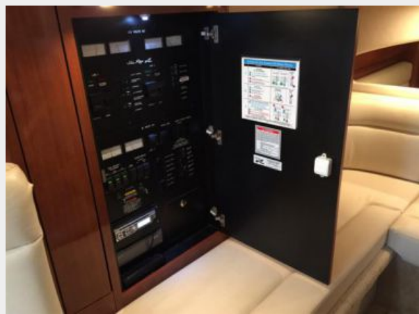
Main Distribution Panel
