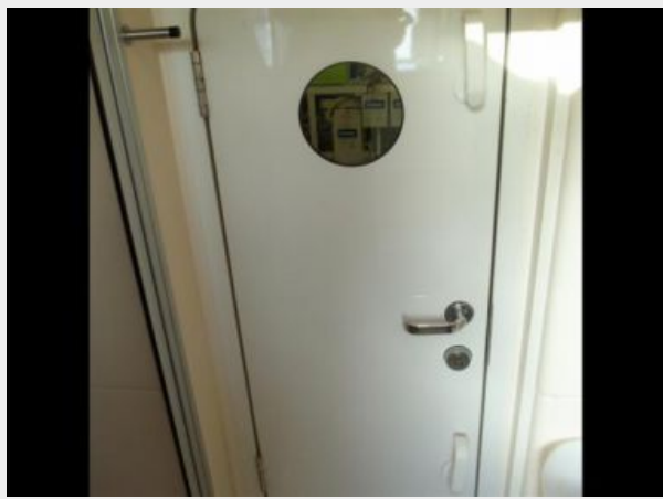
Watertight Engine Room Door
