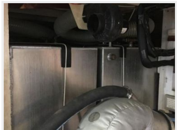
Fuel Tanks Port
