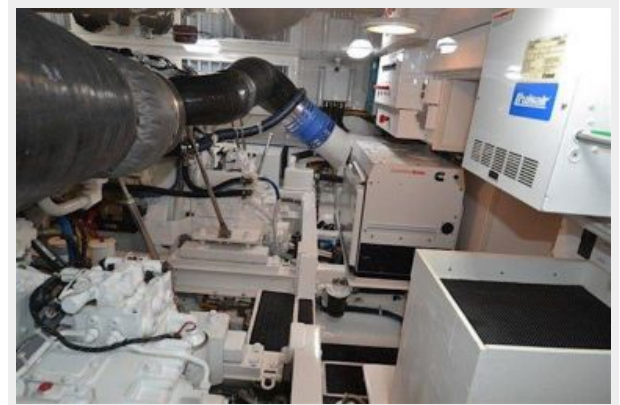
Engine & Mechanical Equipment 8 - Engine Room
