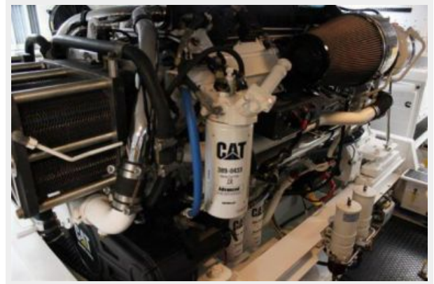
Engine & Mechanical Equipment 6 - Starboard Engine
