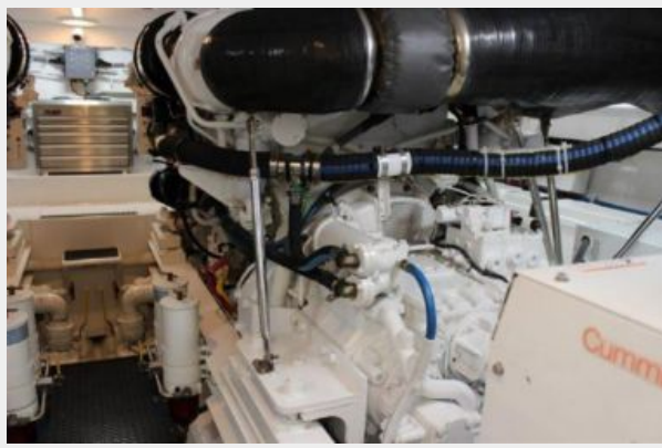
Engine & Mechanical Equipment 5 - Starboard Engine
