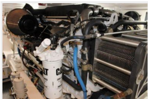
Engine & Mechanical Equipment 3 - Port Engine
