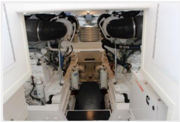
Engine & Mechanical Equipment 1 - Engine Room
