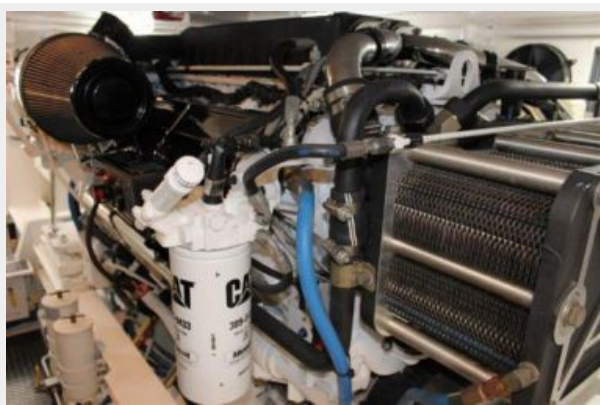
Engine & Mechanical Equipment 3 - Port Engine
