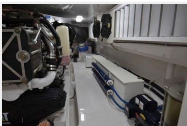
Engine & Mechanical Equipment 9 - Water Maker
