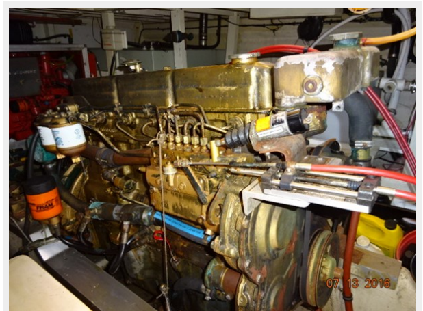
36' Grand Banks main engine photo1
