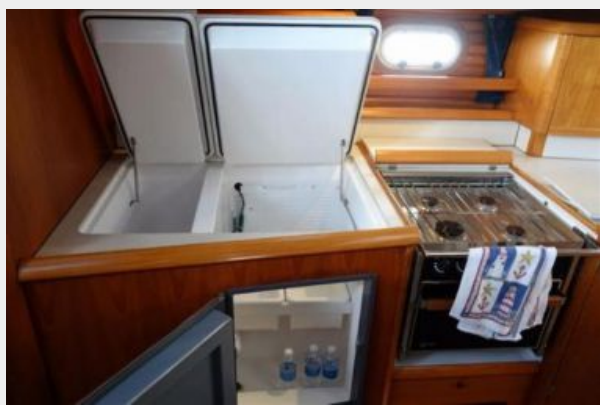
Galley (Refrigeration & Icebox)
