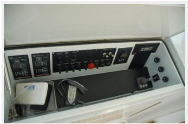
Switch panel compartment, Thruster panel
