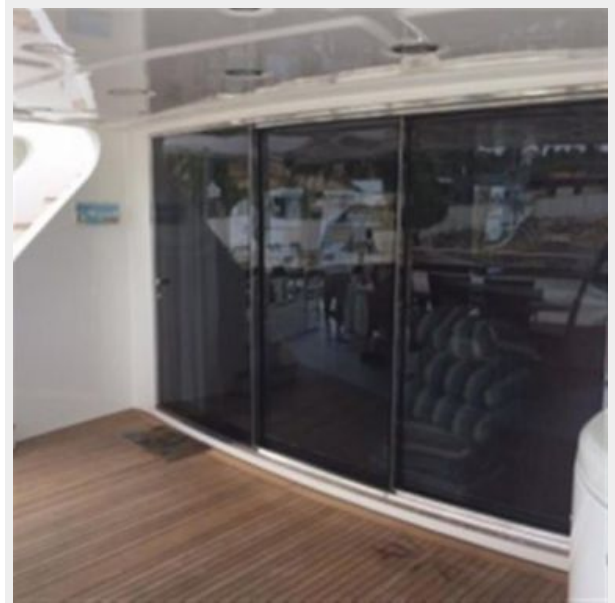
Aft deck entry doors
