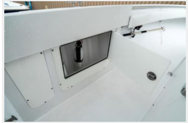
Port Fire Extinguisher
