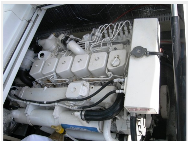
Main Engine Starboard
