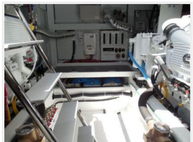
Engine Room Access 2
