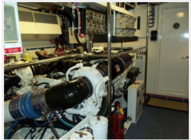
CUSTOM ENGINE ROOM SEALING
