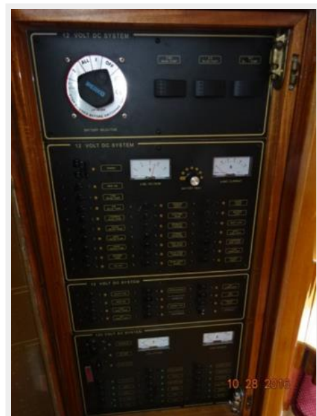
40' Albin electrical panel
