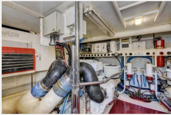
Full Beam Aft Engine Room
