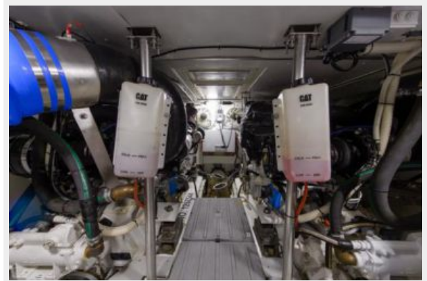
64' Azimut - Engine Room 1
