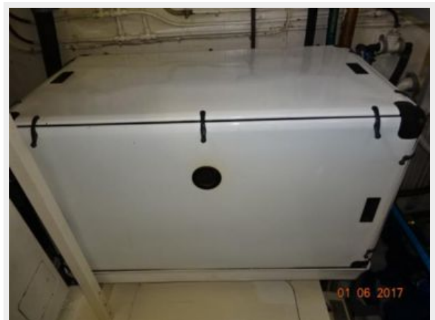
56' Nautical Developments generator soundbox
