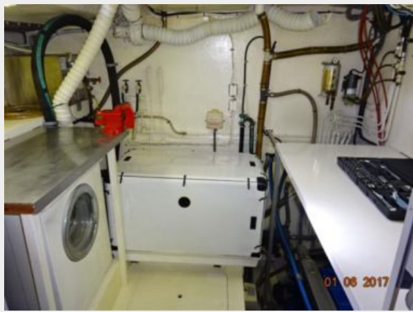
56' Nautical Developments engine room
