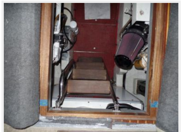
Engine room access ladder.JPG
