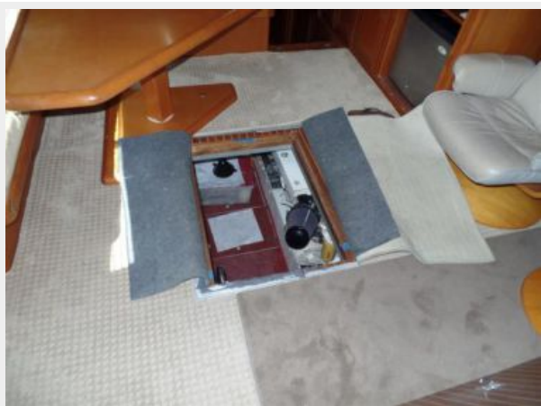
Engine room access.JPG
