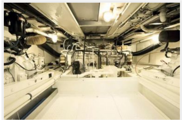
Engine Room Aft
