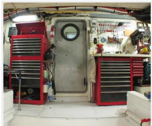
Engine Room Access / Tool Chests
