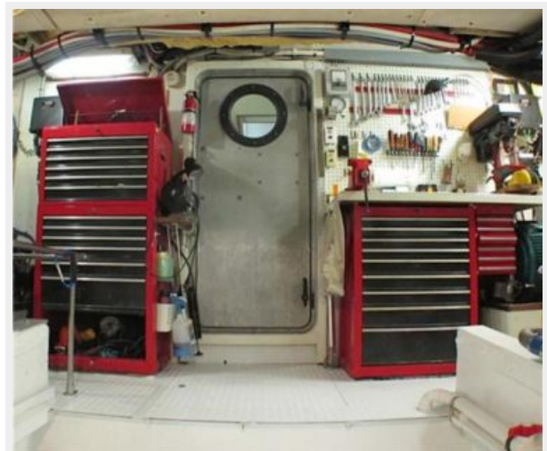
Engine Room Access / Tool Chests
