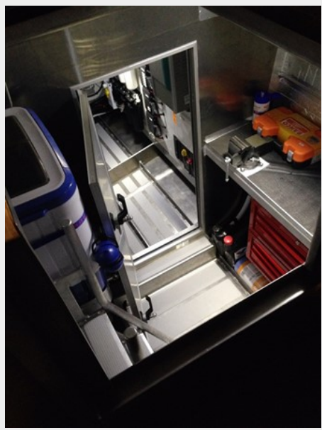
Engine Room Companionway
