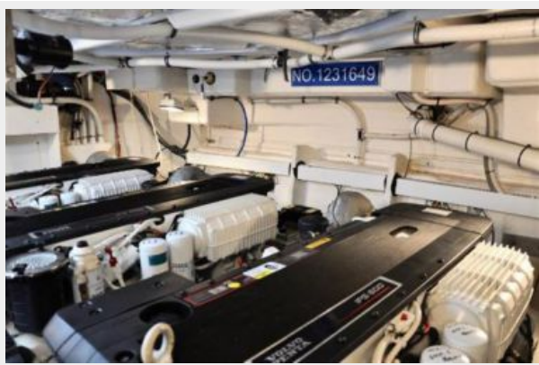
Engine Room Aft View
