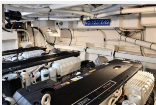
Engine Room Aft View
