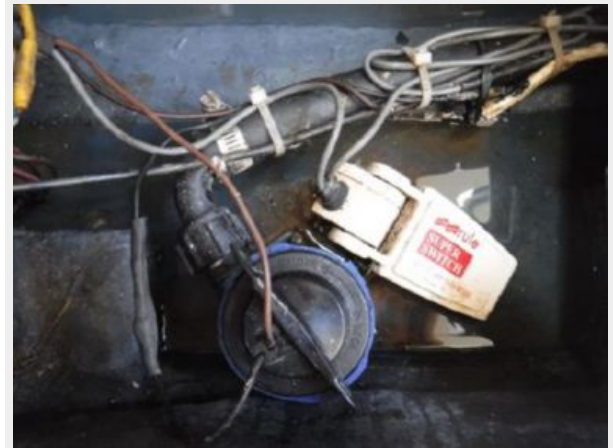
Bilge pump and switch
