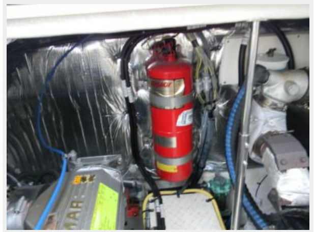
Automatic Fire Extinguisher System
