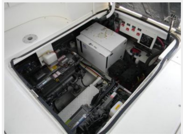
Engine Room Access
