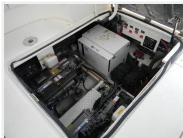
Engine Room Access
