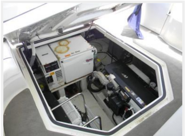
Engine Room Access
