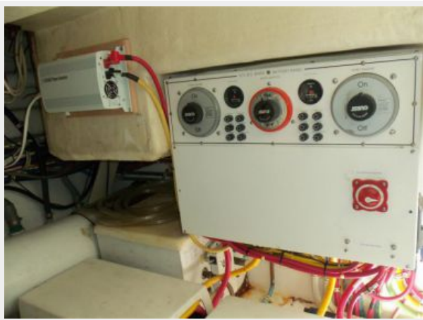
Engine Room Aft
