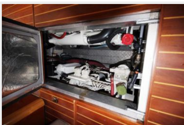
Clean Engine Room
