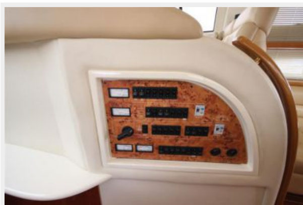
Main Distribution Panel
