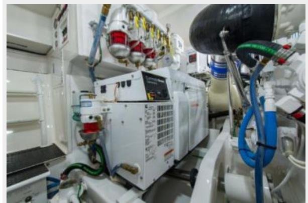
Engine Room Port
