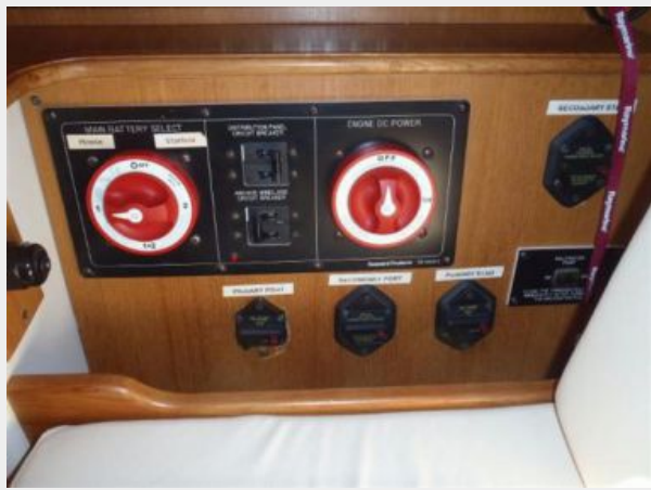
Electrical Control Panel
